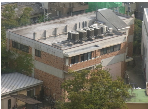
30,000 kW Substation (66kV → 6600V)
